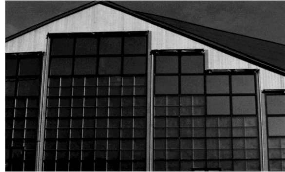
Figure 1-9: Indirect Gain. Shelly Ridge Girl Scout Center, Philadelphia Area Council.
